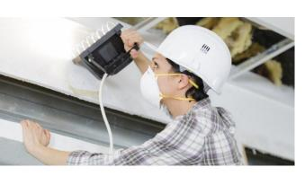
Building tune-ups, also known as retrocommisionings, aim to optimize energy and water performance by identifying low- or no-cost actions related to building operations and maintenance. Building tune-ups assess buildings and implement operational and maintenance improvements to achieve energy and water efficiency such as changing thermostat set points or adjusting lighting or irrigation schedules.
